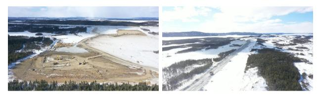
Left. Overburden removal at the future process plant location looking NW with haul road in background. Right, Production haul road under construction, looking SW towards Leprechaun pit. Both February 2023
