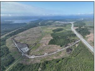
Figure 5: Construction of the Toe Road for the Tailings Management Facility. Advancement of the construction toeroad from the southwest (left) and northeast (right) simultaneously, July 2023
