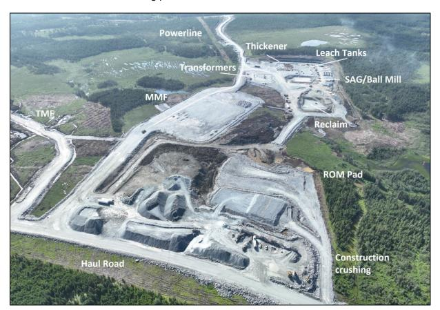
Figure 1: Valentine Process Plant Site, Looking South, July 2023. TMF: Tailings Management Facility, MMF: Mine Maintenance Facility
