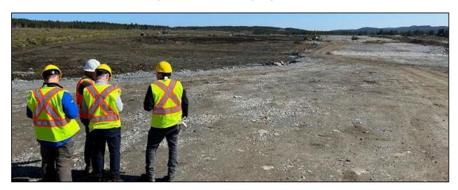
Figure 2: "Zone 6" Rockfill placed on prepared and approved foundation for the TMF Phase 1 Dam, looking northwest. On the upstream side (top left of photograph) shows the prepared foundation without any fill material placement, August 29, 2023.
