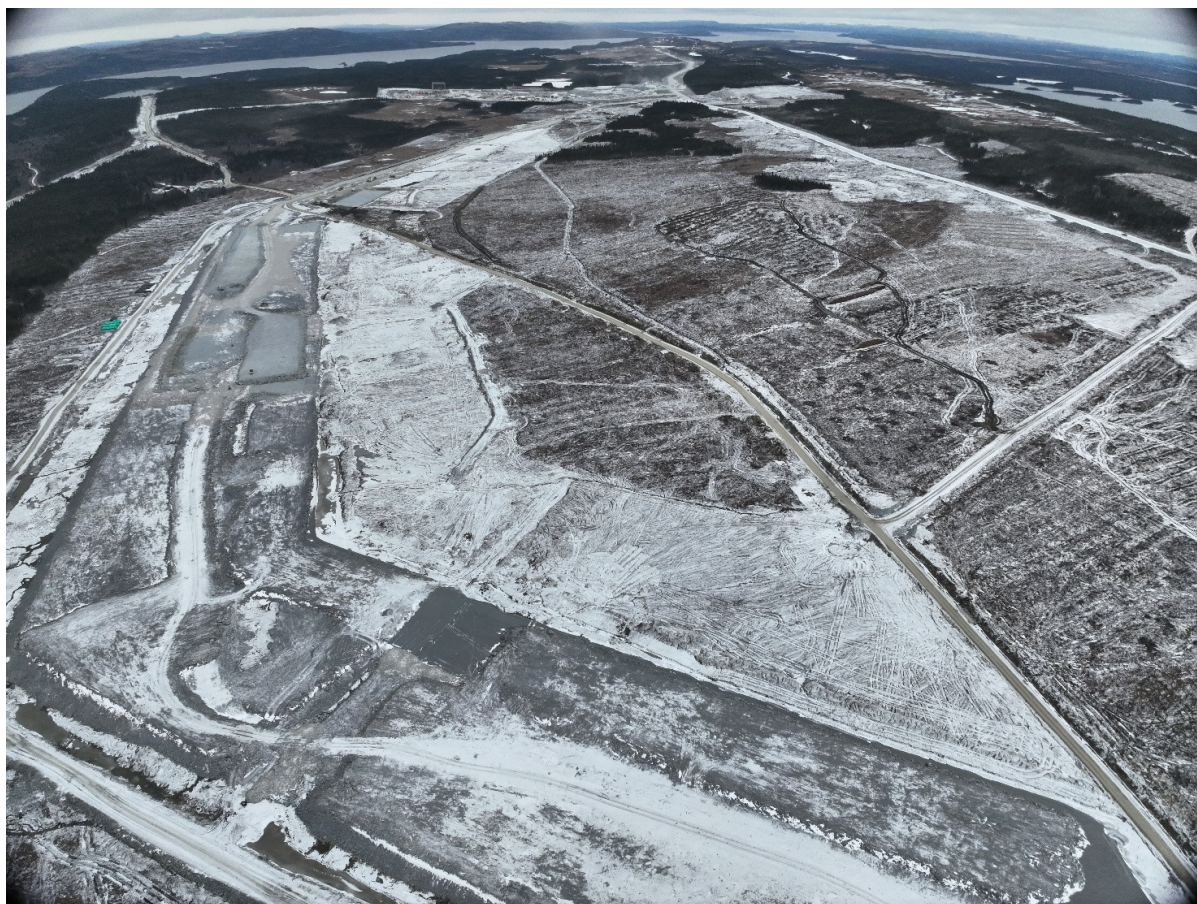
Figure 2: Valentine Gold Project Tailings Management Facility, December 2023
