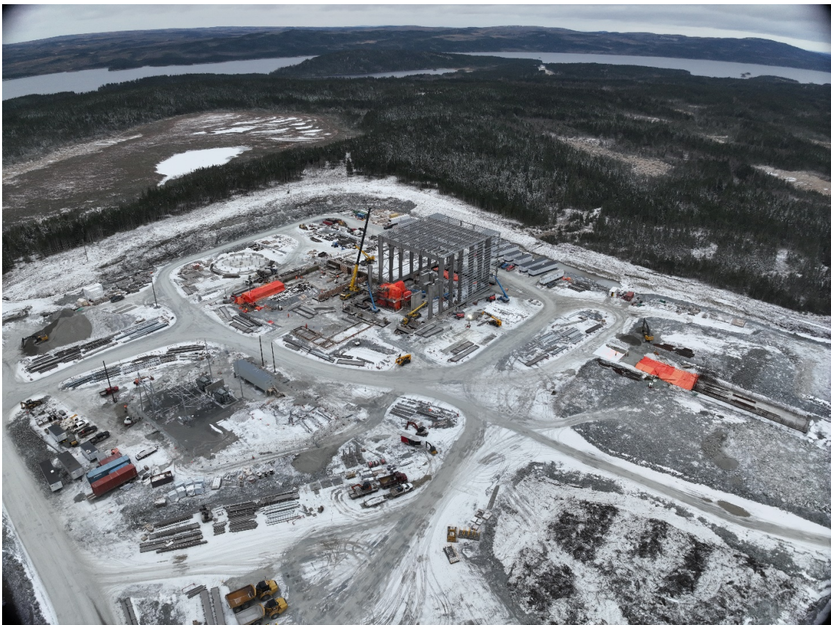
Figure 1: Valentine Gold Project Mill Site, December 2023
